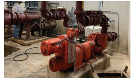
Before installation of new pump
